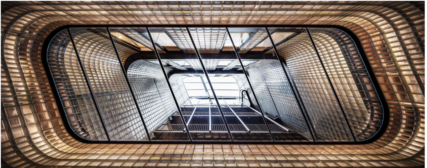
4" Shaped Block, Minimum Radius for 90° Turn
