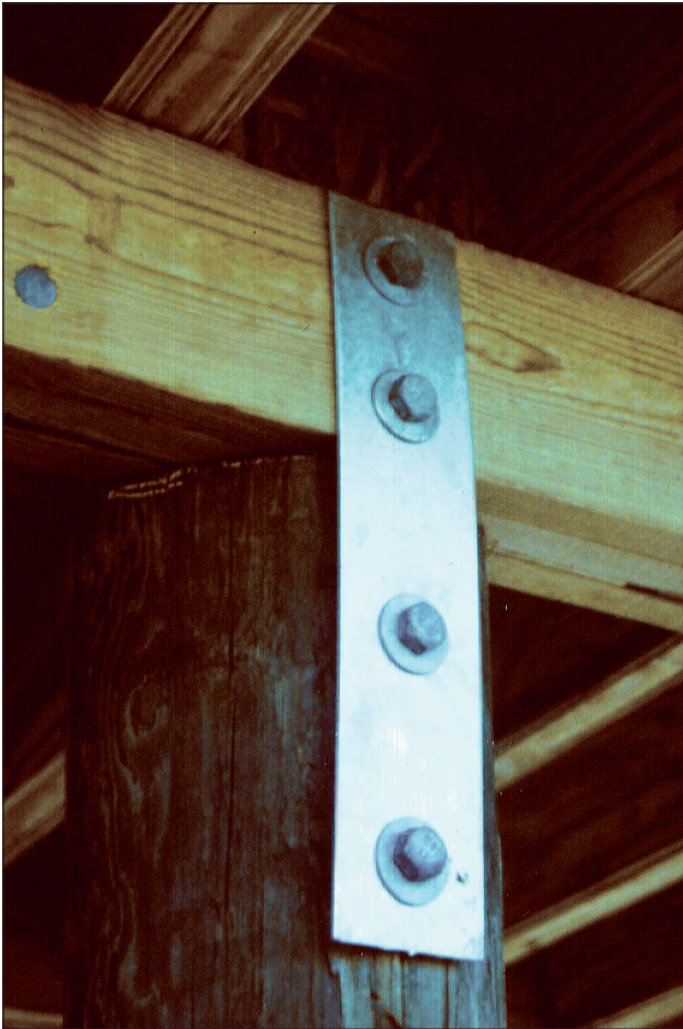
Metals corrode at a much faster rate near the ocean. Always use well-protected hardware, such as this connector with thick galvanizing. (For information about pile-to-beam connections, see Fact Sheet No. 3.3, Wood Pile-to-Beam Connections.)
