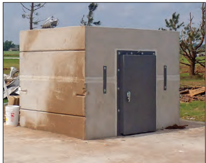
Figure 5-1: Safe room that remained standing after an EF5 tornado (Newcastle, OK, 2013). The photo shows the safe room after the event, after debris had been cleared away.
