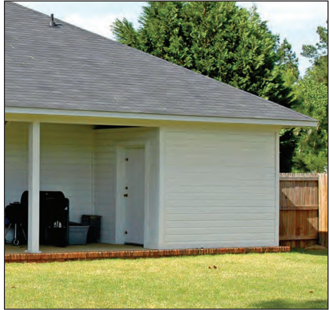
Figure 3-3: An above-ground safe room constructed as an addition to a slab-on-grade home in a way that matches the aesthetics of the home (outside Tuscaloosa, AL, 2011)
