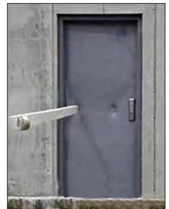
Tornado safe room impact test results: Door assembly passed; no perforation or latch/lock failure
