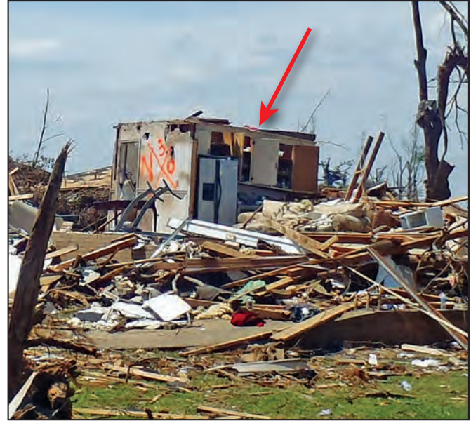
Figure 3-4: Core remnants of homes sometimes survive a tornado as shown in these photographs of site-built homes where a closet (red arrow in left photograph) and a bathroom behind a kitchen (red arrow in right photograph) remained standing after an EF4 tornado (Tuscaloosa, AL, 2011)
