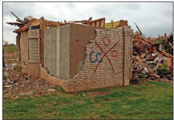
Figure 5-2: Site-built safe room that withstood the impact of the Moore tornado (Moore, OK, 2013)
