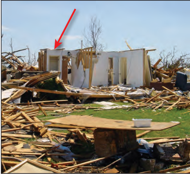
Figure 3-4: Core remnants of homes sometimes survive a tornado as shown in these photographs of site-built homes where a closet (red arrow in left photograph) and a bathroom behind a kitchen (red arrow in right photograph) remained standing after an EF4 tornado (Tuscaloosa, AL, 2011)
